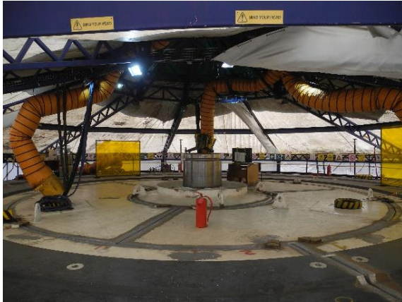
New tub sections aligned and block-welded. Purposely designed temporary shelter Confined space forced ventilation
