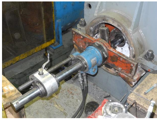
Hoist and drag gear cases alignment check and insitu line boring
