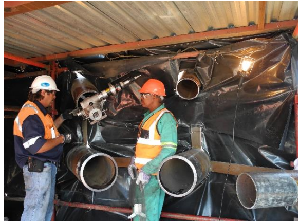
Insitu machining of boom chord and lacing weld preparations during chord replacements
