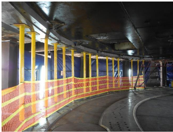
Slew bearing upper rail installation, alignment, drilling and mounting after machining of the support pad
