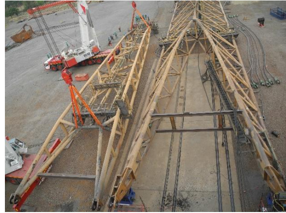
Boom removed - mast removal in progress
