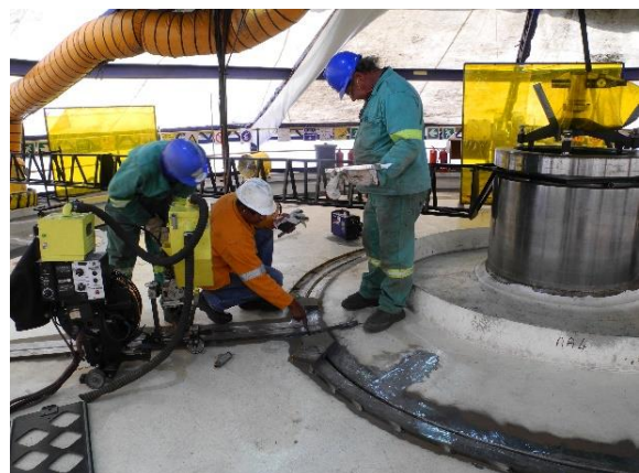
Quality control – alignment and root gap verifications
