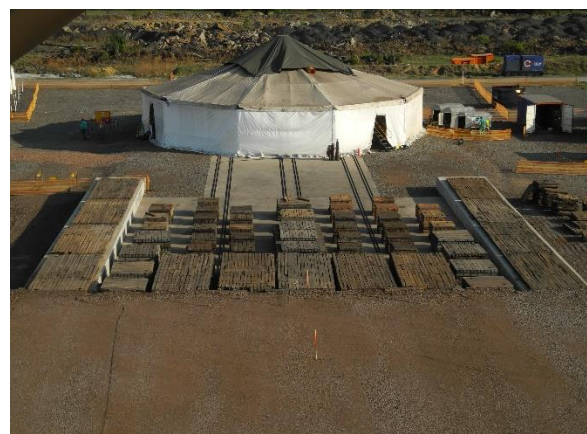
Tub replacement pad – temporary shelter cover the new erected tub
