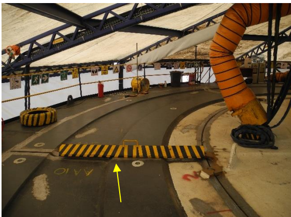
Covers to protect people on-deck from interior gouging and grinding sparks
