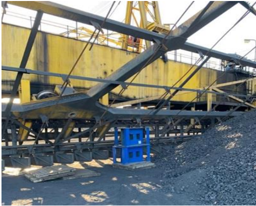
Bridge reclaimer chain and guide replacement
