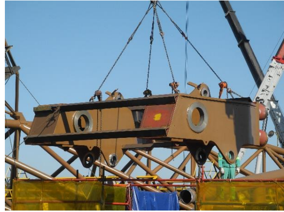
Mast head replacement – new upgraded mast head sub-weldment
