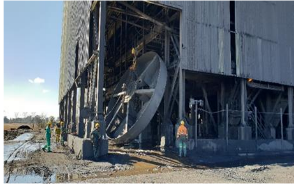
Shale wheel replacement
