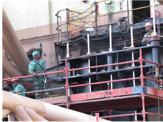
Fairlead mounting bore line boring
