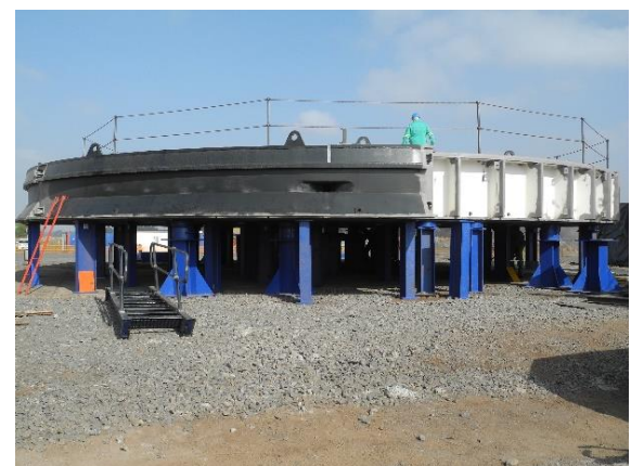
New tub assembling and alignment
