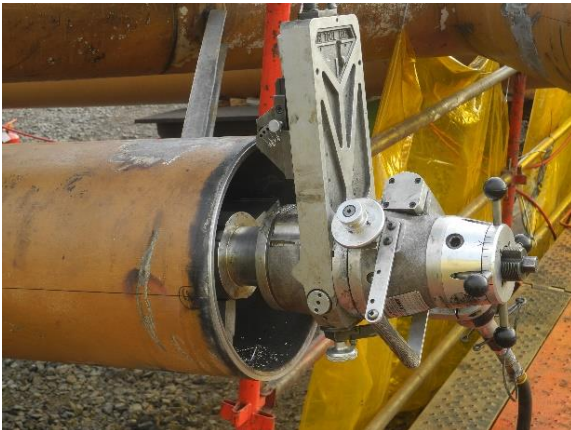
Mast chord machining during mast head replacement
