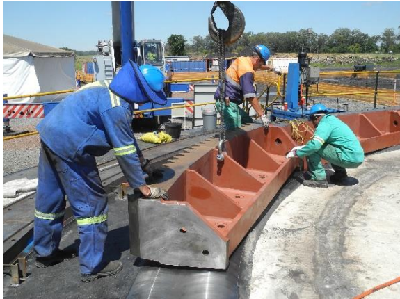
Rack segment installation and alignment
