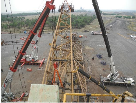
Boom removed - mast removal in progress
