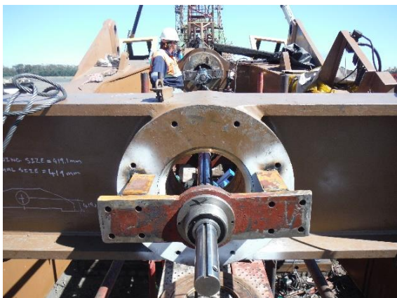
Boom point sheave assembly mounting hub line boring
