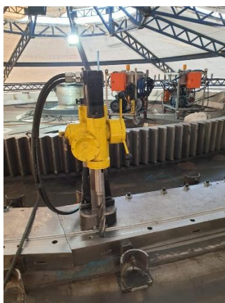
Drilling of lower swing rail mounting bolt holes in progress
