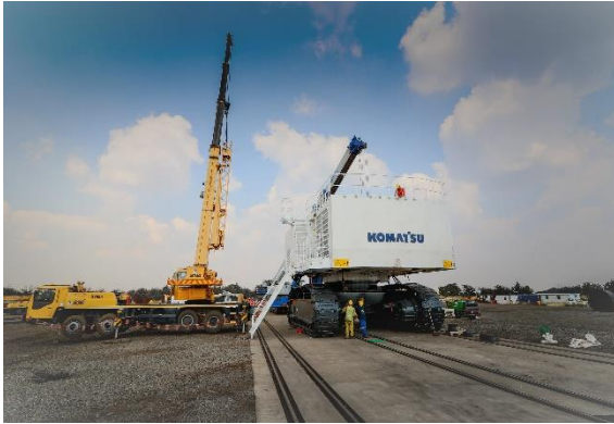
New excavator erections
