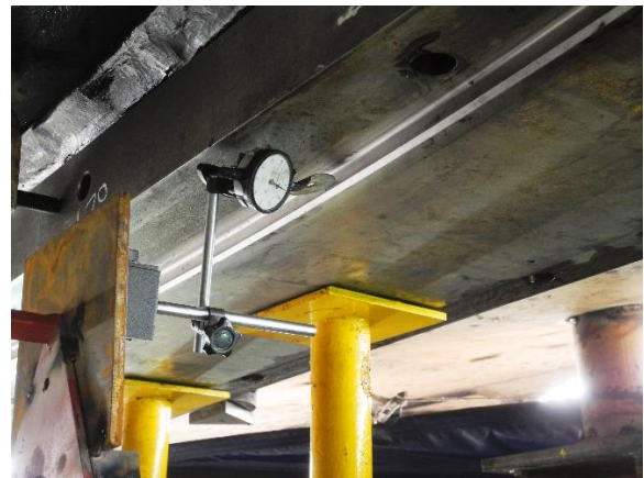
Final alignment of upper rails
