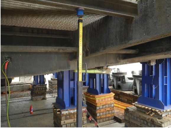
Gauge to monitor machine stability while lifted and supported
