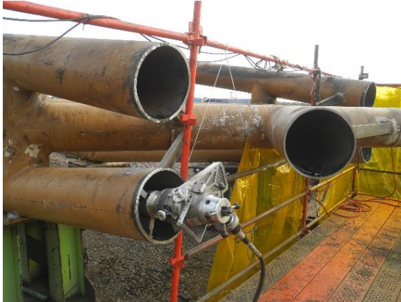
Insitu machining of mast head chords and lacings to accommodate new mast head
